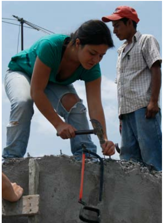
Montessori High School at University Circle, Cleveland, Ohio, X-Term, Oxaca, Mexico, water cistern.
